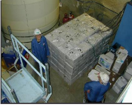
60t tank area in the SNO water utility area
