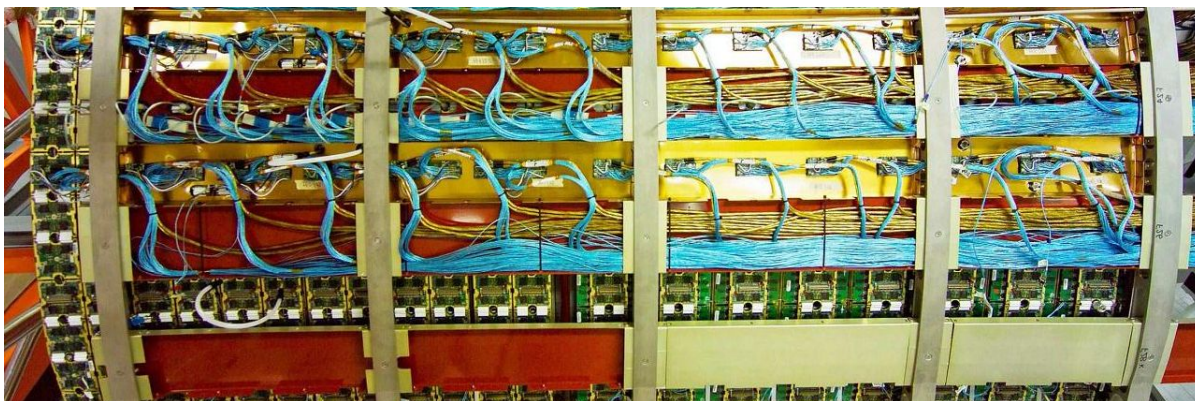
Figure 19. Partially assembled End Cap showing two full cable trays at the top and one empty cable tray at the bottom. Each tray carries cables for 1/32nd of the detector and acts as part of the outer Faraday cage of the detector. The blue cables are the 36 AWG data and control shielded twisted pairs, the heavier orange-brown cables are low-voltage supply cables. The light colored HV cables are just barely visible in the upper tray on the left. In this view the triplet boards serving the A type Wheel nearest the interaction point are on the left and the PPF1 connectors are just out of the picture on the right.
